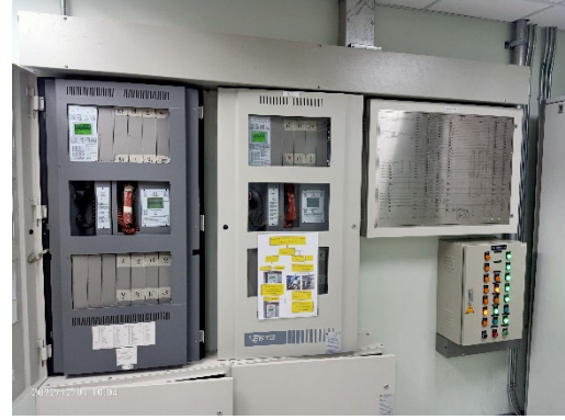
fire alarm control Panel
